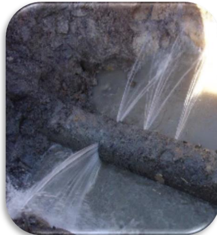
Reducing Inflow and Infiltration associated with Wastewater Infrastructure
