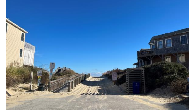
Juncos Street Dune Infiltration
