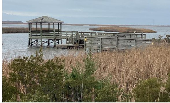
Estuarine Pier Replacement
