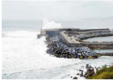
Figure 8.2. Mutriku, Spain, oscillating-water-column-breakwater integration. Source: obs/Voith GmbH
