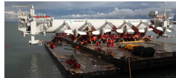
Figure 8.5. Five tidal turbines integrated with the Oosterscheldekering storm surge barrier in the Netherlands. Photo from HydroWorld.com (2015)
