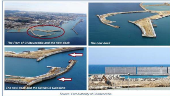
Figure 8.3. The Resonant Wave Energy Converter 3 Device in Civitavecchia Port, Italy. Photos from Maestrale (2017)
