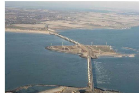
Figure 8.4. Oosterscheldekering storm surge barrier in the Netherlands. Photo from Amazing Planet (2014)
